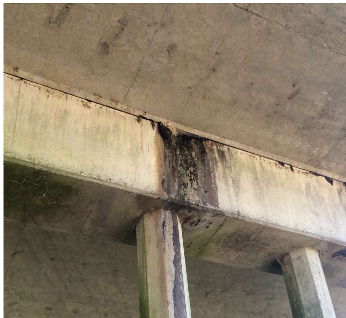
PHOTO 1 Description Bent 3 east face spall
