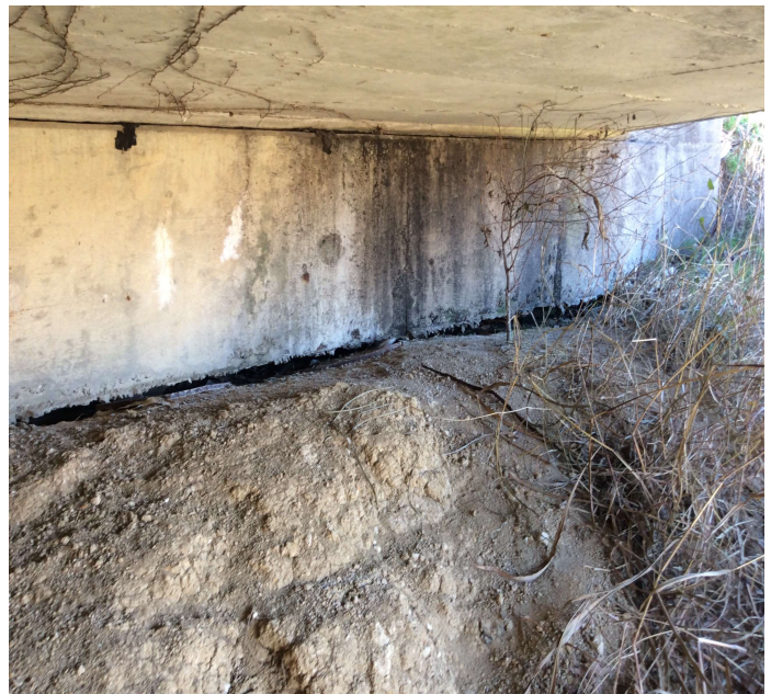
PHOTO 2 Description Erosion under bent 1 cap left side
