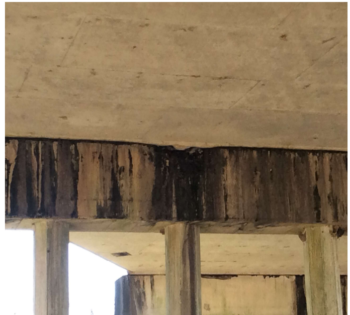
PHOTO 5 Description Bent 4 east face spall over pile 7
