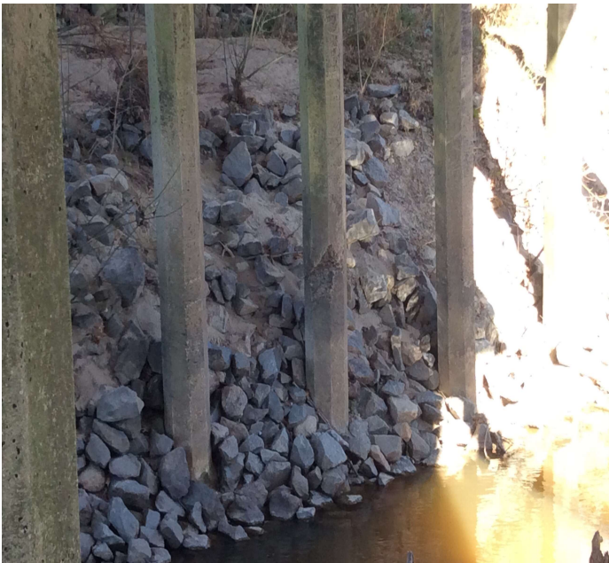
PHOTO 1 Description Bent 5 pile 6 spall near ground line
