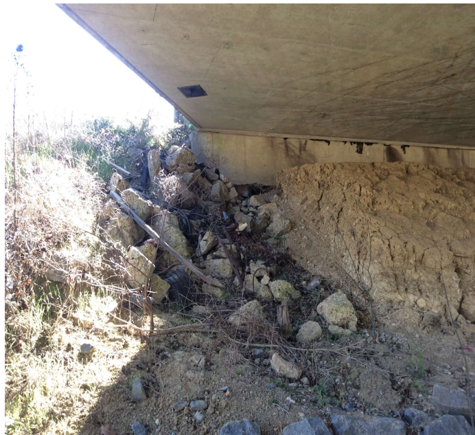
PHOTO 1 Description Erosion under bent 1 cap and in span 1 right side
